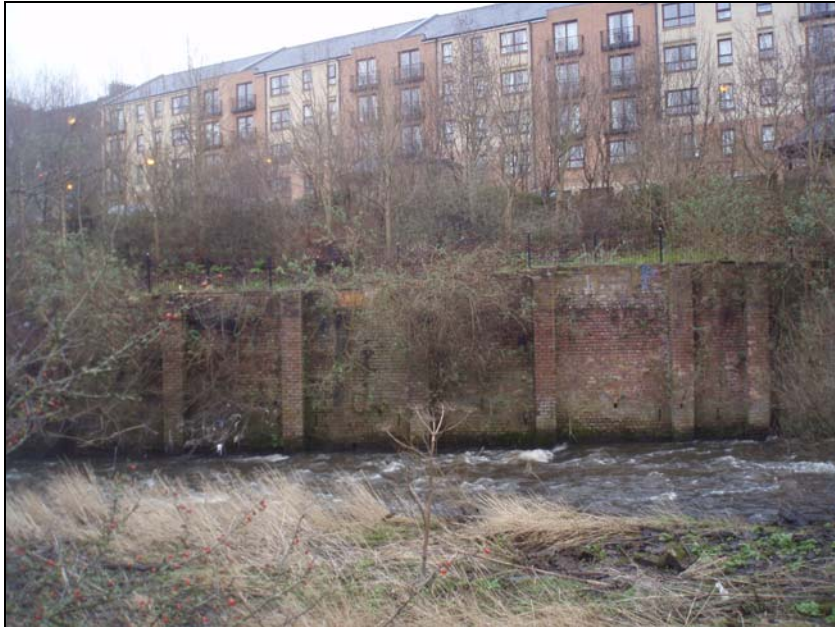
Photo 2: The retaining wall at the river's edge.
